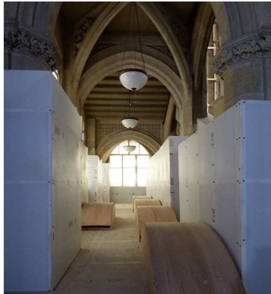
The delicate interiors of the town hall have been covered to protect them from damage during the works
