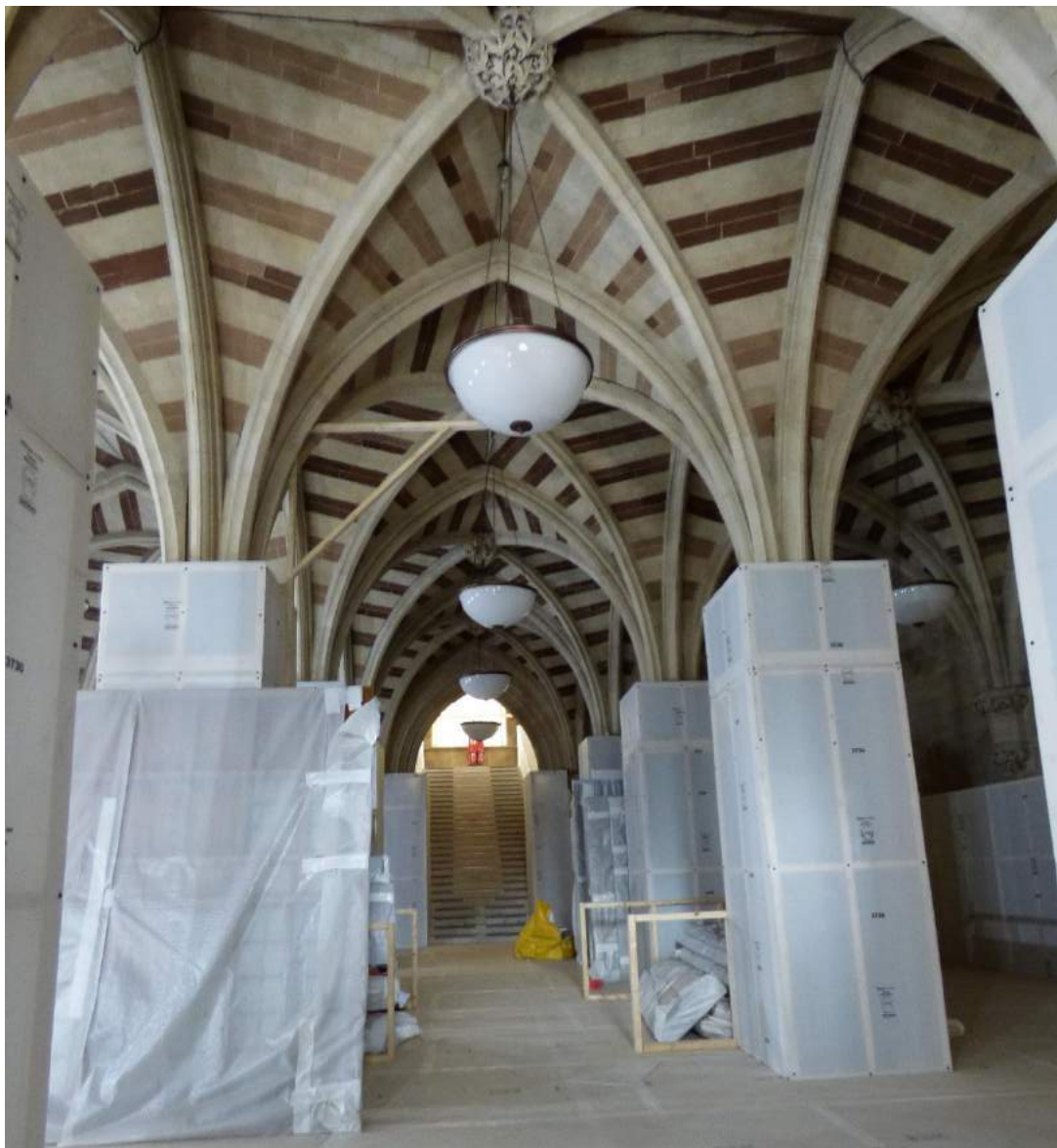
The delicate interiors of the town hall have been covered to protect them from damage during the works
