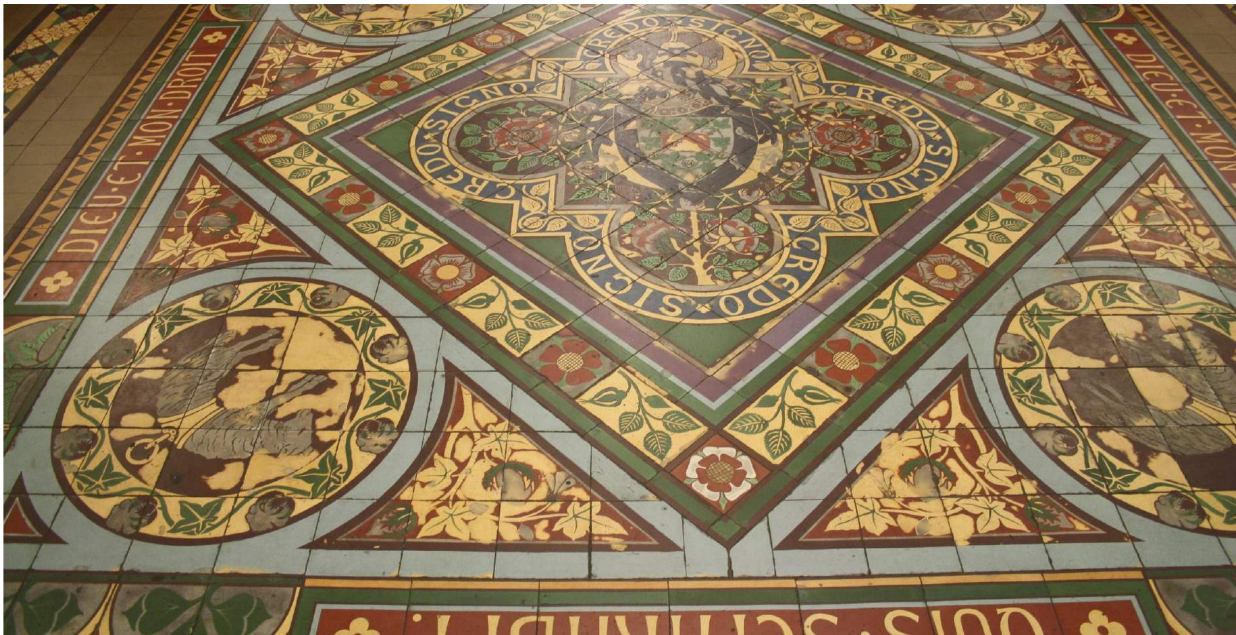
Example of the minton floor tiles which are showing signs of wear and tear and will need cleaning. A protective layer will be added to prevent further deterioration in the future.
